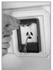
8. Dress extra cable into the hole (or wall box if used) and position the camera, starting at the top onto the plastic back frame.
