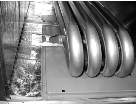
FIGURE 14 - DISCHARGE PANEL IN PLACE
