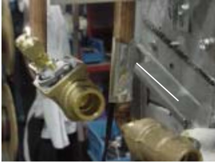
Figure I-MR-3. Attach the changeover sensor to the entering water pipe as shown for changeover to work properly
