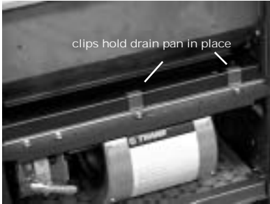
Figure M-MP-3. To remove the main drain pan on vertical fan-coil units, disconnect the clips holding the pan to the fanboard.
