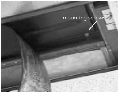
Figure M-MP-4. To remove the main drain pan on horizontal fan-coil units, peel the insulation from the edges of the pan's underside to access the mounting screws.
