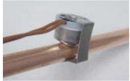
Figure I-MR-7. Electric heat lock out switch installed
