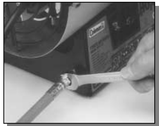
Tighten with Wrench
