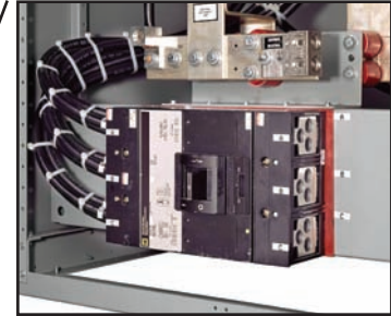
Fig. 12: Ground and neutral disconnect links
