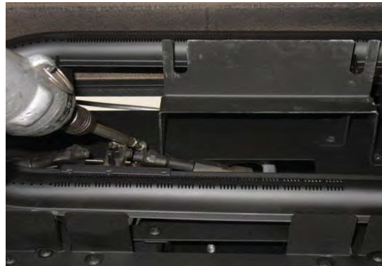
Installing Mid Log Bracket
