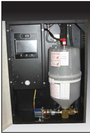
Hinged door provides full access for service.
