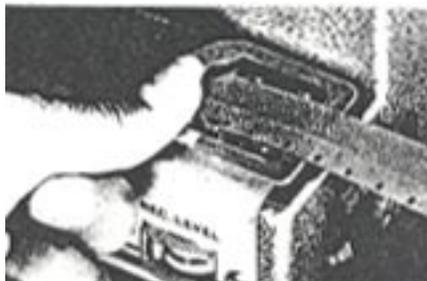
1. Insert film in trimmer and cut with raised end.
