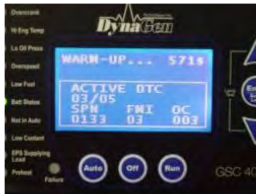
Figure 14 – Five active DTC messages and the 3PrdP one being displayed
