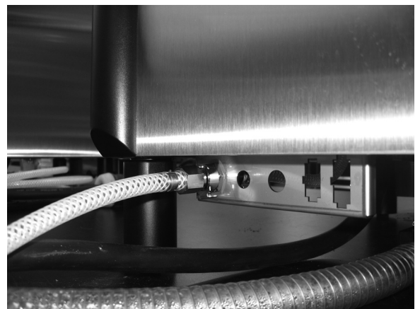
INSTALL WATER SUPPLY LINE
