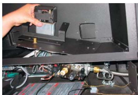
Diagram 5: Lift out Valve Tray Assembly
