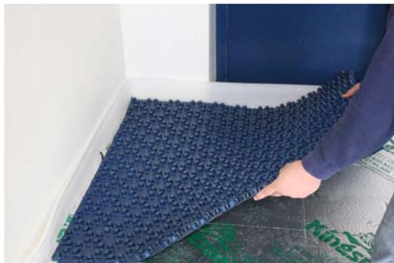
Take the next template and position it on top of the first one with the cut outs in the same position and press into place.
