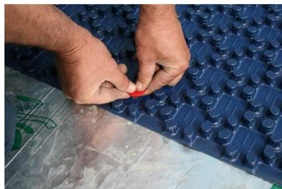
When all the templates have been fitted the heating pipe is simply 'walked in' in line with the CAD or design and is then after pressurising and testing is permanently covered by screed.
