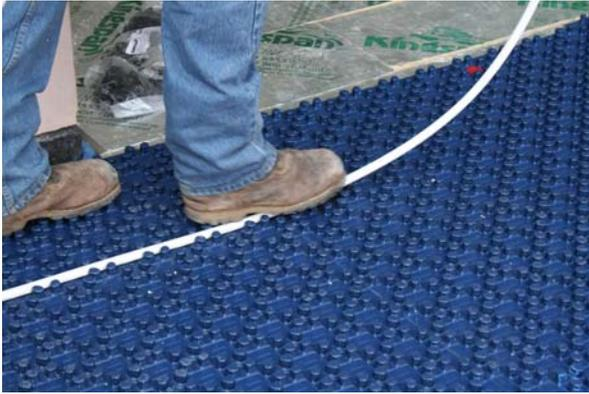
The ecotherm floor templates hold the pipe against movement when screeding. Optimum screed depth is 65mm from panel base.
