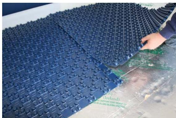
Fix the templates to the insulation using red plastic nails or staples.
