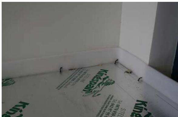
**IMPORTANT:** If you are going to use a liquid screed you need to use an expansion strip with a thin polythene strip attached to it.
