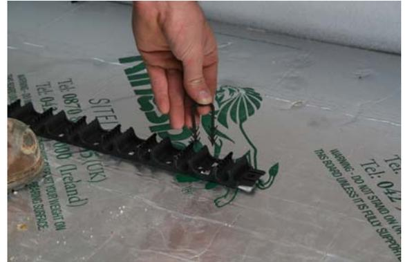
**Figure 12 Pipe work should then be fixed into the grip rails.**
