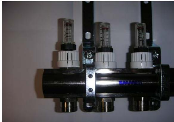
**Step 1** Lift up the white cap so it covers the flow gauge nut as in fig 29 below.
