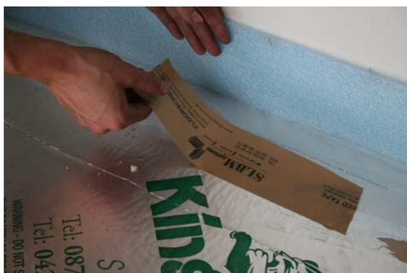
This polythene strip must be taped to the membrane that has been laid on top of the insulation with specialist floor screed tape in order to ensure a watertight seal.
