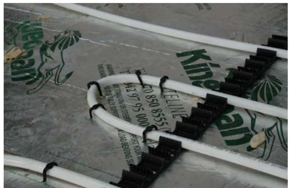
When fixing to grip rails keep the coil laid flat on the floor and roll it out in front of you. Alternatively, a second person can roll out the pipe ahead of you whilst you fix the pipe.
