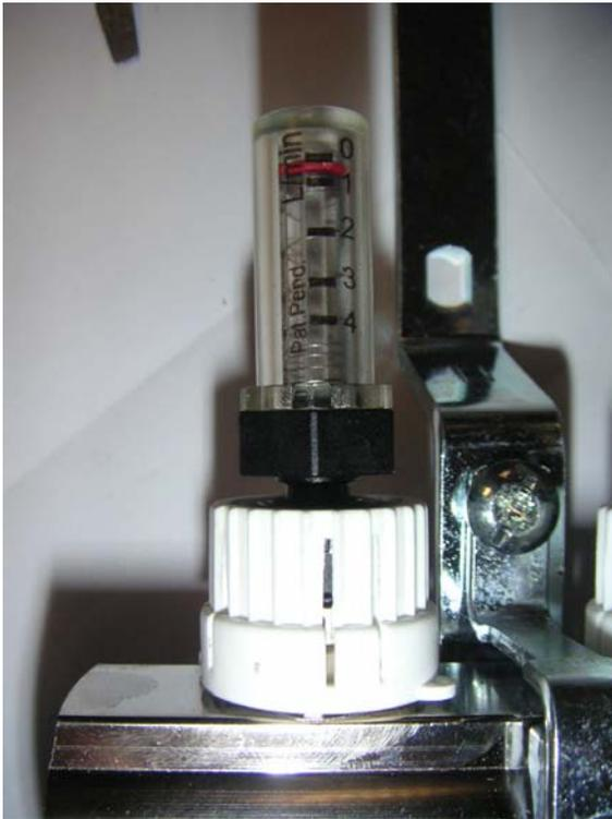
You can now twist the flow gauge clockwise or anti-clockwise which adjusts the flow rate when the under floor heating system is in operation. For the time being leave the flow adjuster about halfway between the highest and lowest position.
