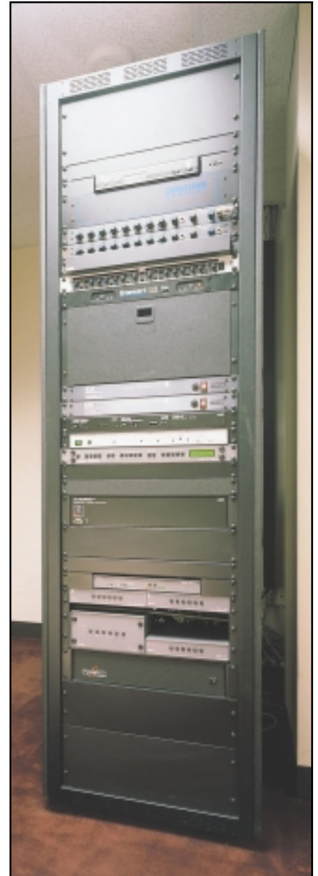
EXTRON'S SYSTEM SWITCHER, SWITCHERS, AND SCAN CONVERTER IN THE A/V RACK
