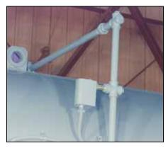
Figure 1-7 Auxilary Low Water Cutoff
