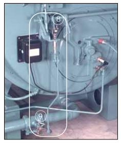
Figure 2-13 Gas Modulating Cam, linkage and Butterfly Valve
