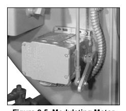
Figure 2-5 Modulating Motor
