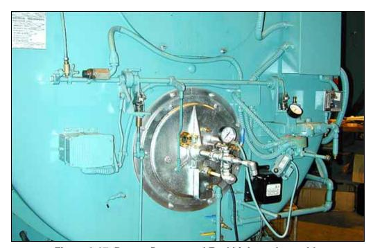
Figure 2-27 Burner Drawer and Fuel Linkage Assembly
