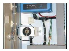
Figure 2-1 Gas/Oil Selector Switch
