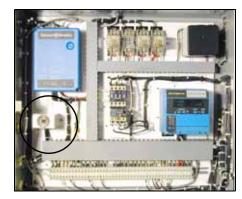
Figure 2-21 Control Panel with Gas/Oil Selector Switch
