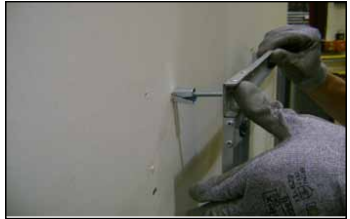
Figure 4.6 Installing Anchors in Hollow Wall
