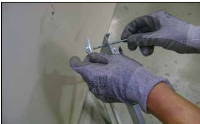
Figure 4.5 Toggle Bolt Installation through Mounting Bracket
