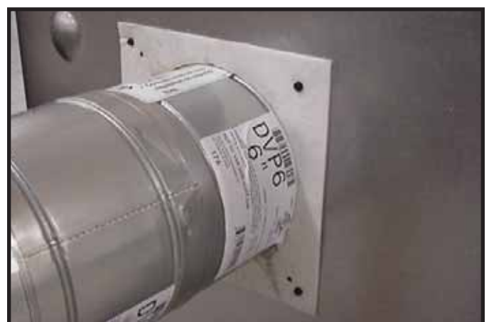
Figure 7.12 Attach the first vent section (it will snap into place). Slide the insulation gasket onto the vent section, up against the appliance and over the tabs. Use two self-tapping screws to secure gasket to outer wrap.
