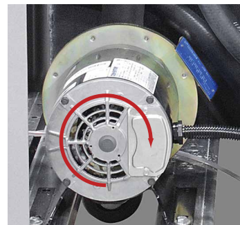
Correct shaft rotation is clockwise.
