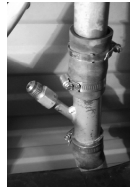
Figure 7: Installing 'Return to Tank' assembly
