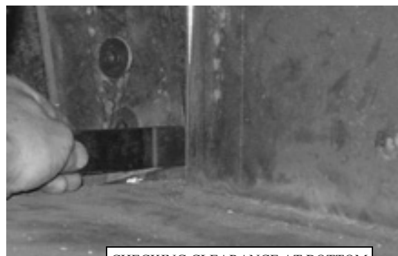
CHECKING CLEARANCE AT BOTTOM OF KNIFE ASSEMBLY
