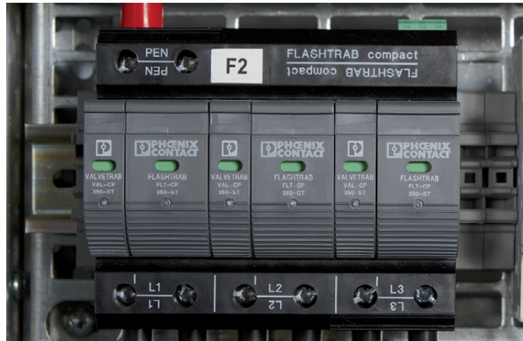
FIG. 5 LIGHTNING CURRENT AND SURGE ARRESTER
