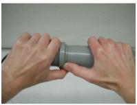
Then, open the plastic tube between the socket joint carefully.
