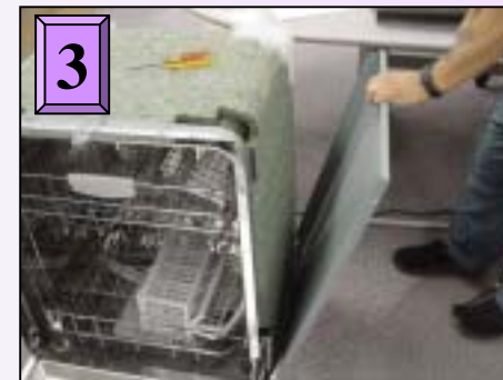
Removing side panels
