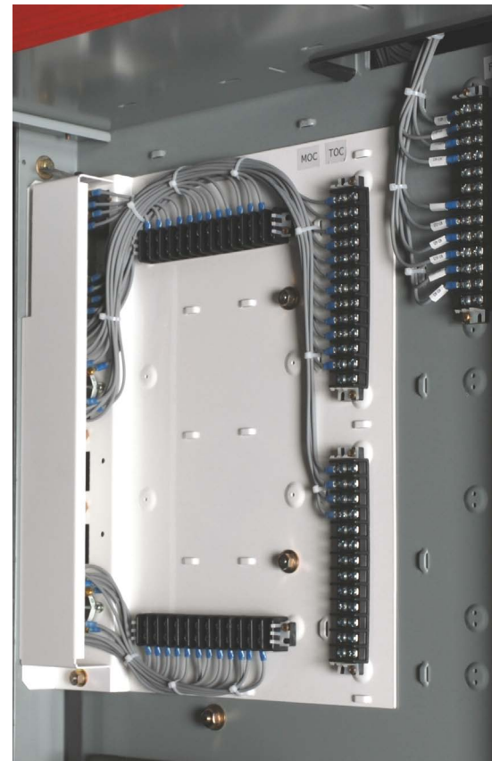
Figure 24: MOCs (12 stages shown) and TOCs (8 stages shown)
