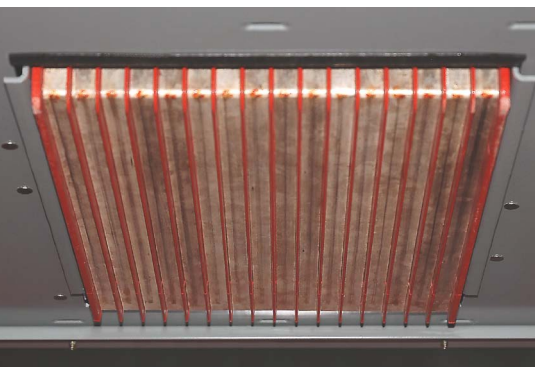
Figure 22: Secondary disconnect (cell portion)
