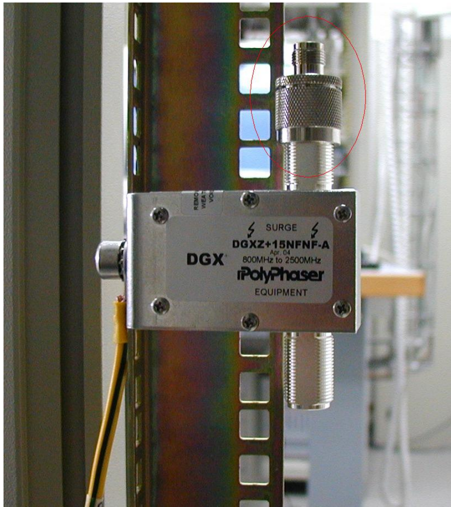
Figure 2-7: Connecting the TNC to N-type Adaptor
