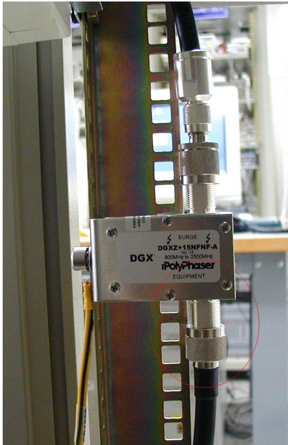
Figure 2-8: Connecting the RF TNC-type side to the “Equipment” side
