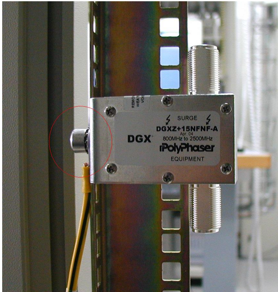
Figure 2-6: Installation of Lightning Arrester on Mast
