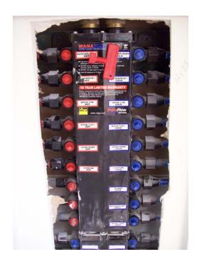
This is the disconnect box for your water heater tank in the attic. You can also disconnect this at the mani-fold system panel, but it is a good idea to disconnect here as well if someone is working on the tank itself:
