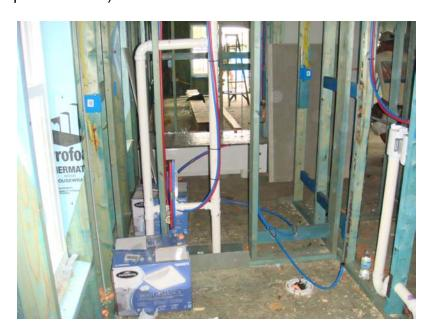
Washer plumbing installed, with red (hot water) and blue (cold water) hoses and white water pipe for filling and draining:
