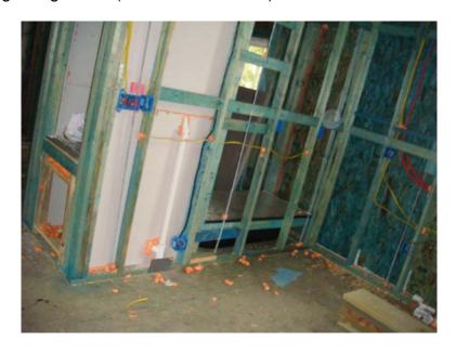
Master and main bathroom plumbing (white water pipes, red hoses for hot water and blue hoses for cold water to sinks and showers), as well as electrical wiring (yellow wires) and boxes (blue receptacle outlets):
