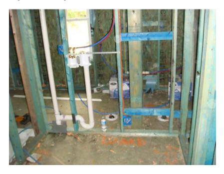
This is your mani-block plumbing distribution system, with red hoses holding hot water and blue hoses holding cold water for each individual plumbing fixture. The main water line comes from below the house (the blue hose coming from the bottom center of the unit), where it is distributed at this point:
