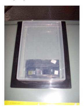
In the case of an emergency, your energy recovery ventilator's disconnect is simply a plug in the attic next to the unit itself:
