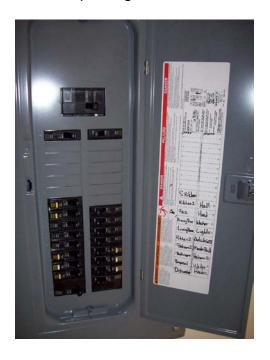
If an outlet or device is still not working, flip the appropriately labeled breaker in your outside electrical panel on the side of your home. Again, if signs of a fire hazard occur, do not switch back into the "on" position:
