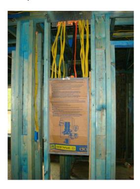
Electrical wiring installed (yellow wires with blue receptacle outlets and switch boxes) with kitchen plumbing on right side (red and blue hoses):
