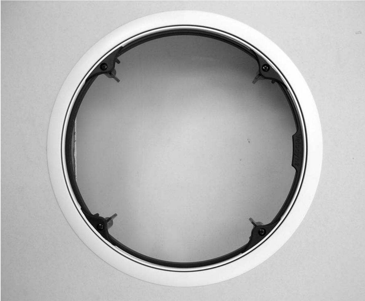
Figure 3. Install the basket flange into the cut-out ceiling material.
