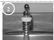
Screw the white quick connect adaptor into the blue female hose. Connect the adaptor to the faucet by sliding the white sleeve down while sliding the connector onto the faucet adaptor.
