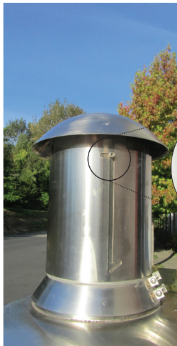
Flue collapsed.
