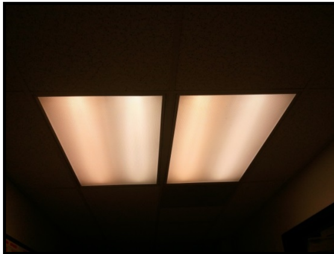
Mismatch of T8 color temperature (Kelvin) in troffer
