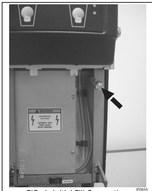
FIG 1 Initial Fill Connection
