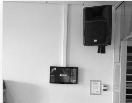
*Installation with a visible installation on the wall with the power supply hidden above the ceiling*
