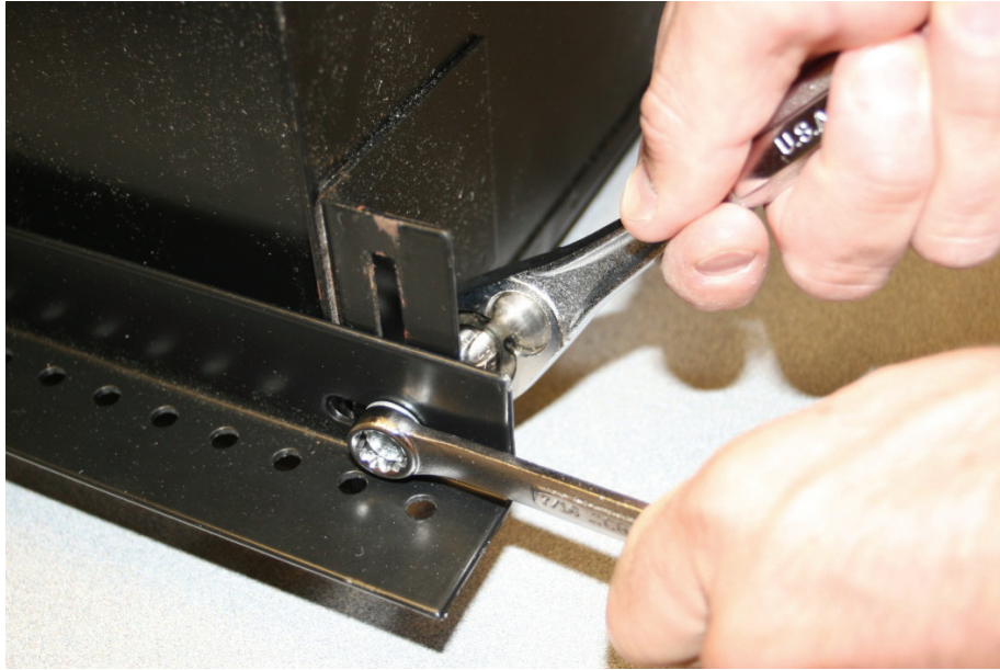
Figure 22: Tightening the rail kit to the backbox
