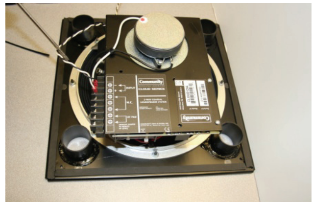
COMPLETED STRAIN RELIEF
