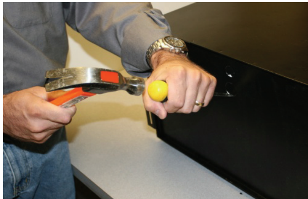
Figure 13: Knocking out the knockout with a hammer and punch
