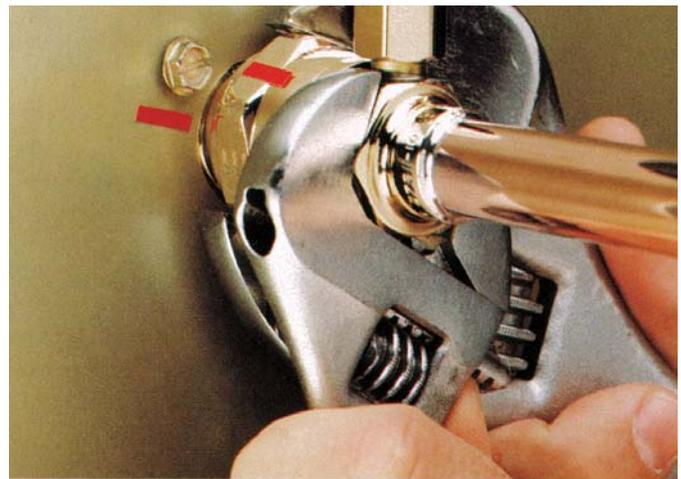
6. After all connections have been made, and after the receiver outlet valve has been opened (do not open yet), check the couplings for leaks.
