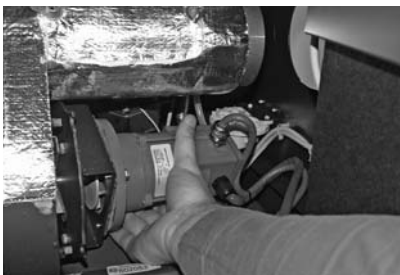
Fig. 101 Removing wing nuts, removing the blower unit
