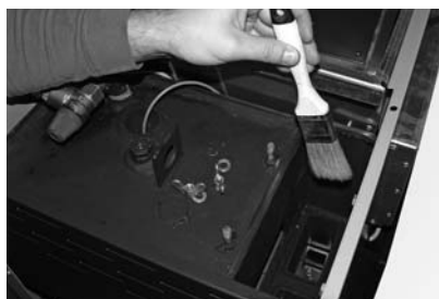
Fig. 92 Cleaning top heating surfaces and linkage
