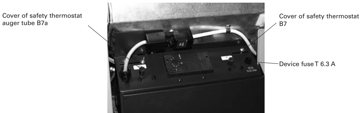
Fig. 109 FireWIN control panel, rear right side panel removed
