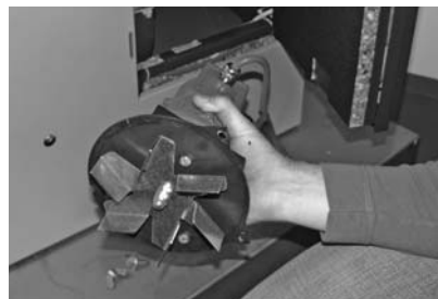
Fig. 102 Cleaning the blower wheel
