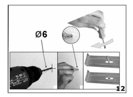
**12)** Using a 6 mm drill bit, drill out two holes on the pencil markings that you made in step 11. Insert raw plugs into the holes and then use a screwdriver to secure the fixing bracket to the wall.
