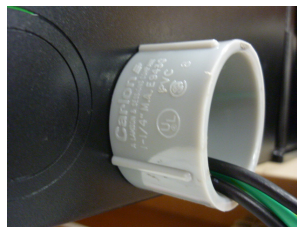
Figure 7.2.2.2: Insert the AC cables through conduit
