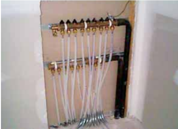
Figure 16: Typical Radiant Floor Header System
