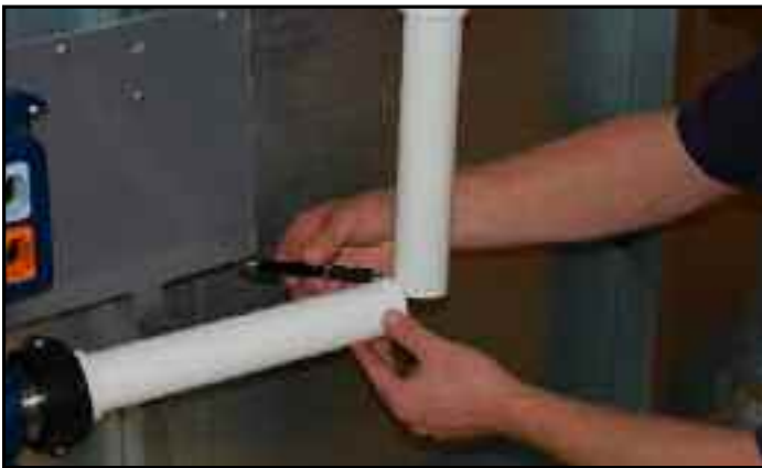
Make a mark on the return assembly stub pipe.
