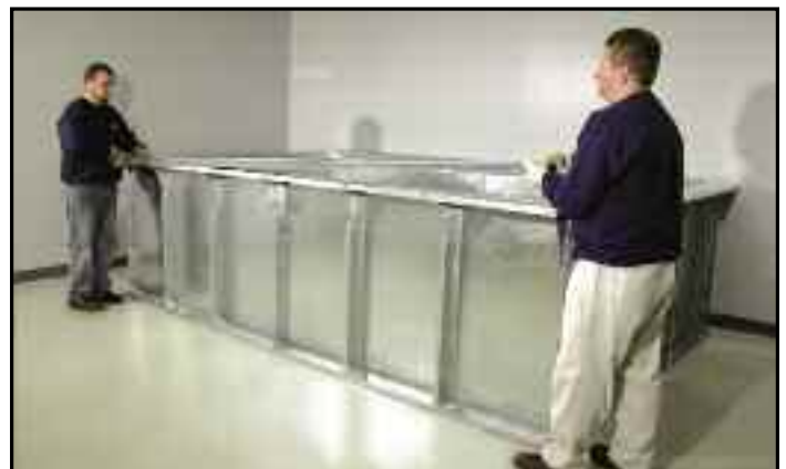
Installing the structural channels.
