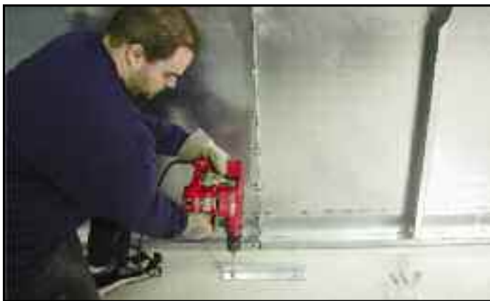
Drilling through foundation to secure blocking angle.
