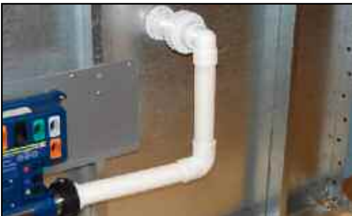
When the flexible PVC pipe and the return assembly has been cut to fit, glue the pieces together.
