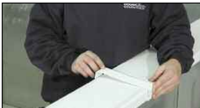
Installing the aluminum cover strip.
