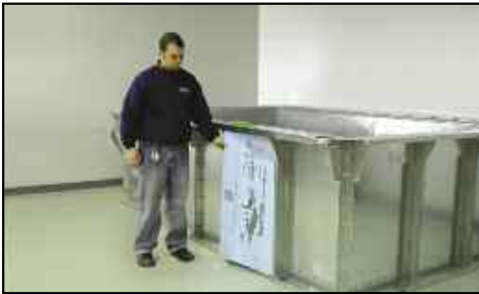
Rigid foam insulation being installed between the support struts.
