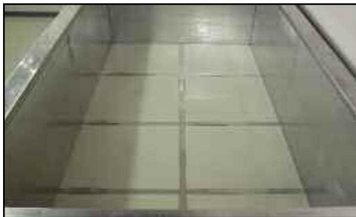
Tension straps in place under pool.
