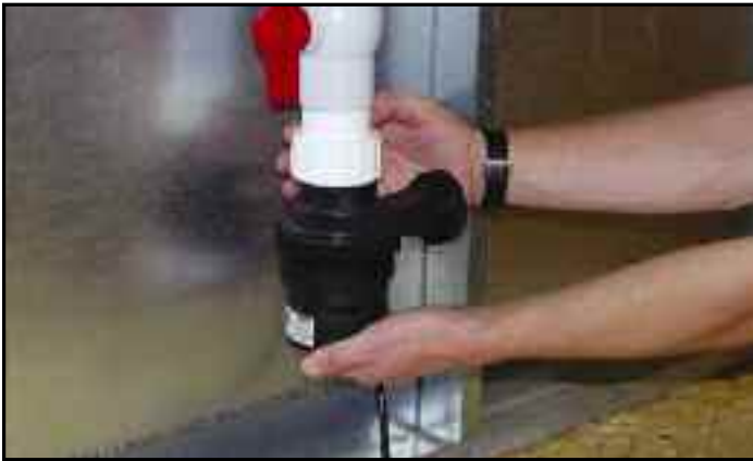
Firmly thread the pump to the skimmer assembly union nut.
