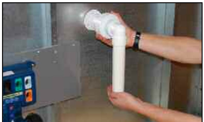
Reconnect the union half to the union half of the return assembly.
