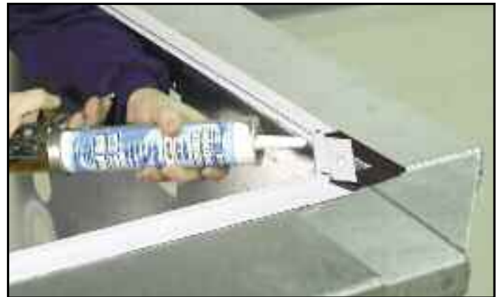
Caulking the liner hanger on the bottom.
