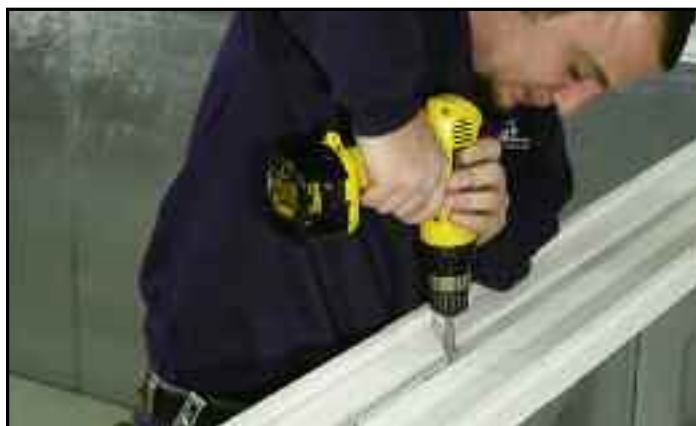
Securing aluminum coping system with tek screws.
