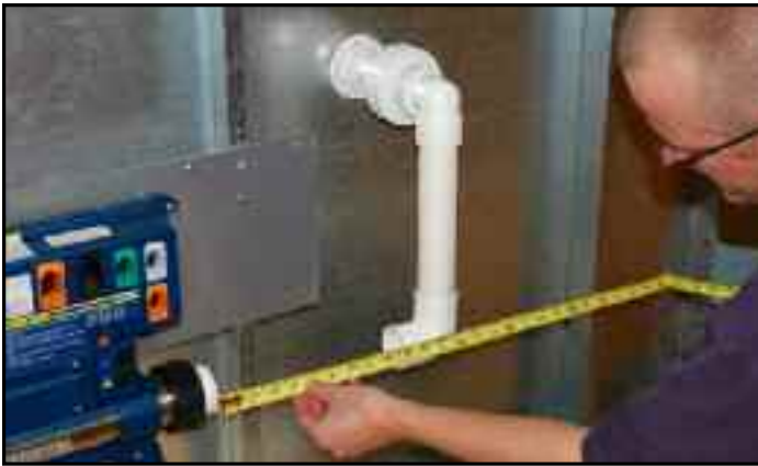
Take a measurement between the elbow and the heater union half.
