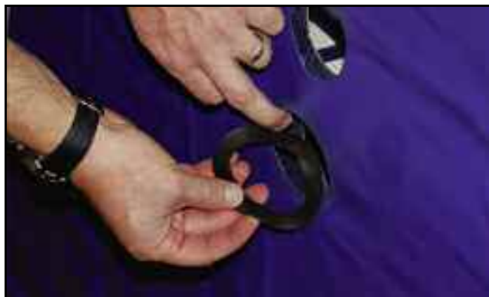
Install one rubber washer between the liner and the pool wall.
