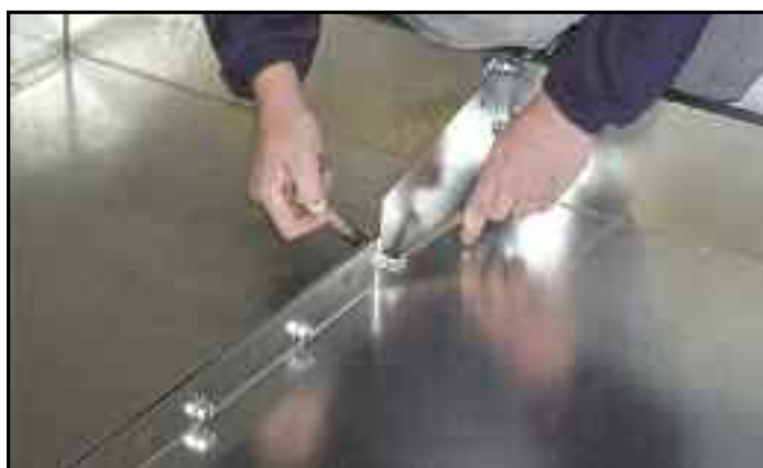
Long side end flanges bolted together with a gusset.
