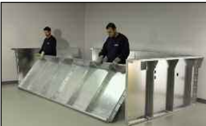
Completing pool enclosure. Note cut-outs on front panel.
