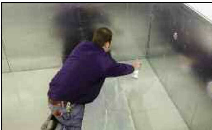
Installing foam with spray adhesive.
