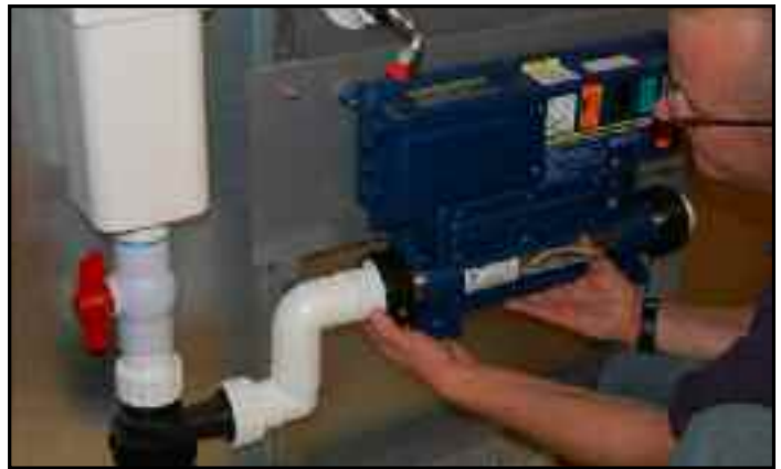
Hold the heater and thread the pump heater connector onto the heater.
