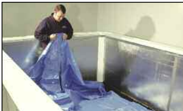
Spread out the liner inside the pool enclosure.
