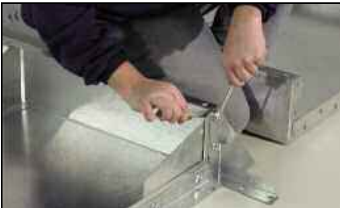
Loosely bolt together the corner angle, top corner angle, gusset and panel.
