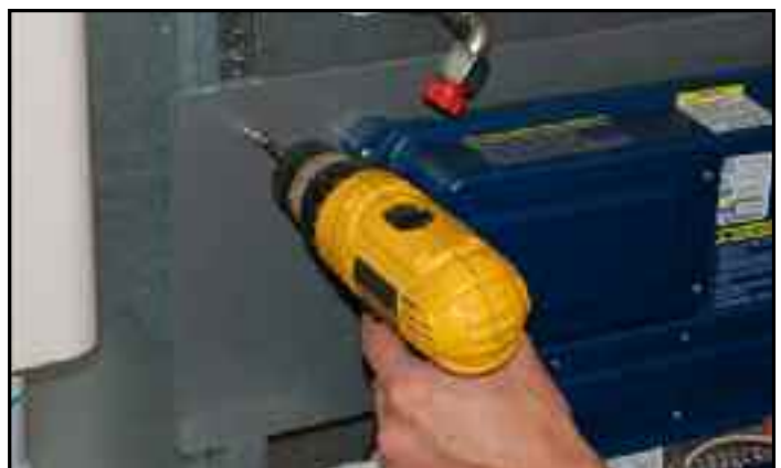
Attach the support bracket directly to the panel Z-braces.
