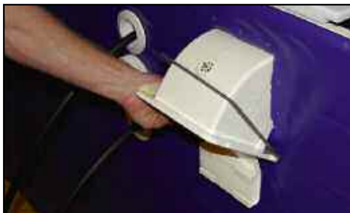
Position the skimmer into the opening of the panel.
