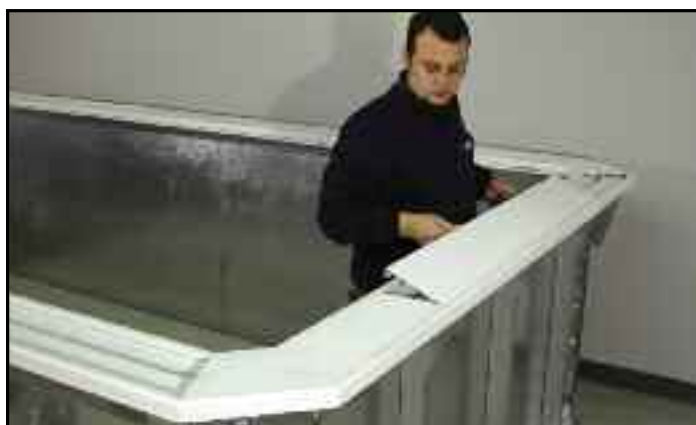
Installing the aluminum coping snap strip.
