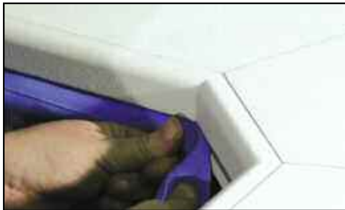
Inserting the liner in the corner of the liner hanger.
