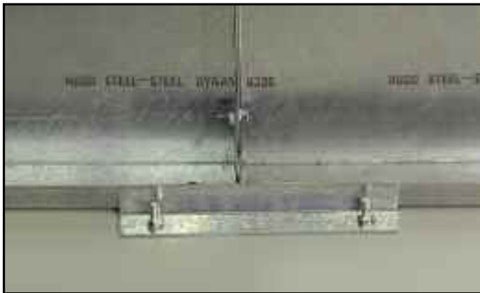
Blocking angle installed with pool panel pushed flush against it.
