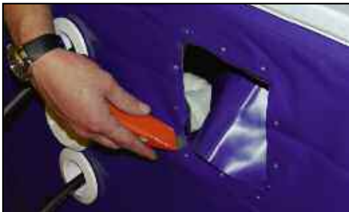
Cut the liner using the skimmer opening in the panel as a template.
