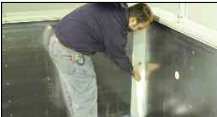
Secure the foam corner inserts with caulk
