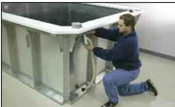
Tape off all thru-wall holes and place vacuum hose through skimmer.
