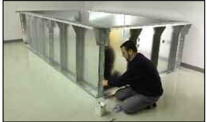
Bolting the pool enclosure together. Note cut-outs on front panel.
