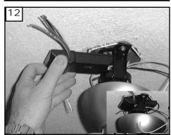
Install remote receiver by sliding into opening in the Mounting bracket. Make sure that the dip switches on the Transmitter and the Receiver are set to the same position. See Fig 38 for remote operation
