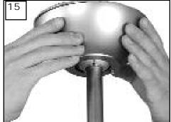
Raise the canopy up and align the two holes in the canopy with the two holes in the hanger bracket. Secure with two screws provided.
