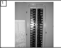
Before you begin installing the fan, Switch power off at Service panel and lock service disconnecting means to prevent power from being switched on accidentally. When the service disconnecting means cannot be locked, securely fasten a prominent warning device, such as a tag, to the service panel.
