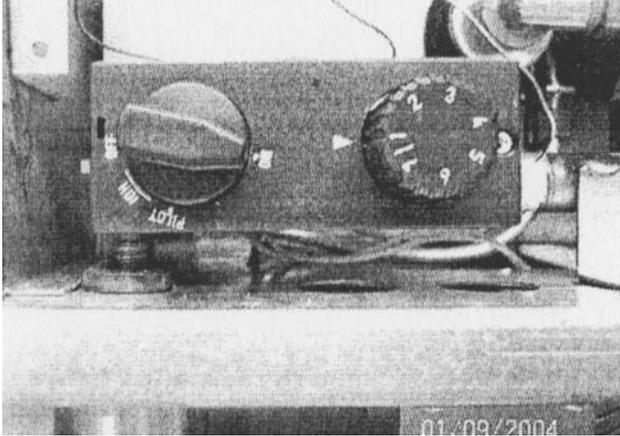
**NOTICE:** When turning on the gas at the propane tank, turn gas on very slowly. Turn valve just a small amount. This allows the gas to get into the lines without shutting the tank regulator down. The regulator on the tank should have a safety feature that is designed to sense a leak. After lighting pilot, open tank valve a few turns.
