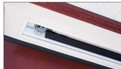
Bottom panel off during installation
