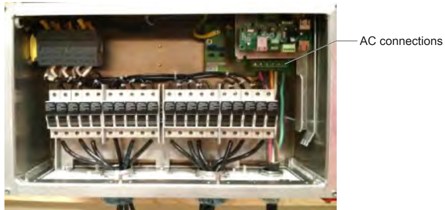
Figure 4-12. 500 V series AC connections
