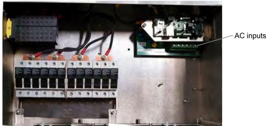
Figure 4-13. 1000 V series AC connections
