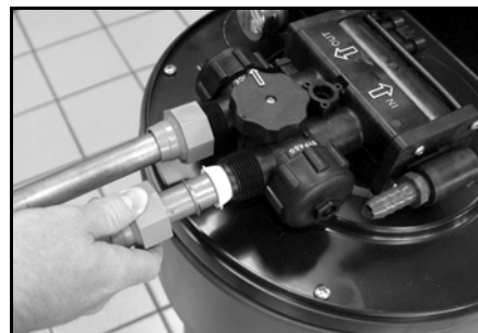
Figure 3: Connect Water Lines. Note the Bypass Valve.
