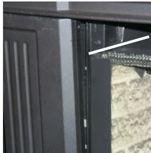
Slide side filler bracket into gap between glass and fire box.
