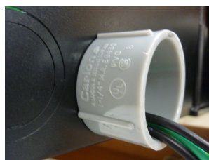
Figure 7.2.2.2: Insert the AC cables through conduit
