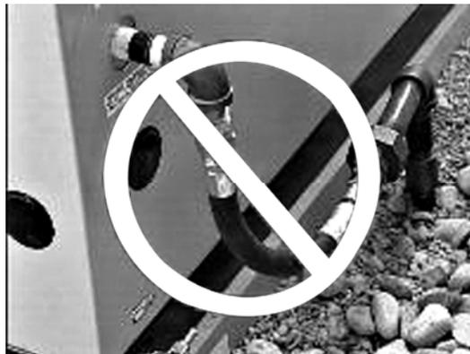
**Figure 5.4 — Incorrect Routing of Flexible Hose**
