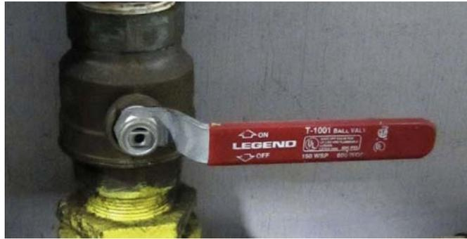
**Figure 5.2 — Full Flow Shutoff Valve**
