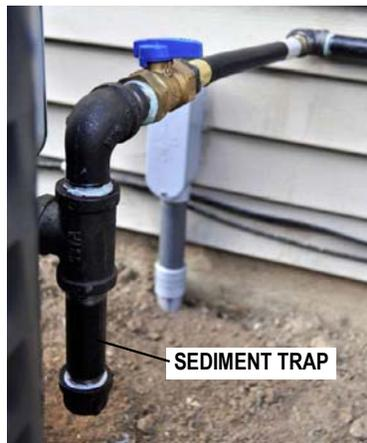
**Figure 5.3 — Sediment Trap**
