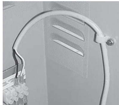
Fig. 2-5, Input Power Cable Clamp
