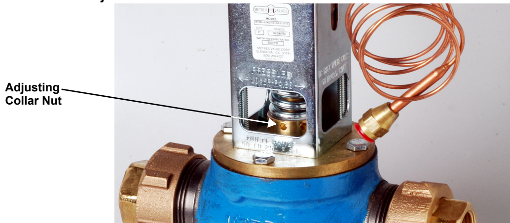
Figure 5 Metrex valve adjustment
