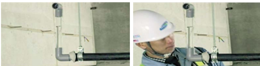
Check for leakages after 24 hours.
