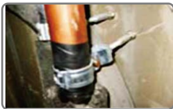
Fixing with a circular band
