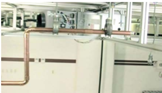
Nitrogen substitution for prevention of copper pipe corrosions
