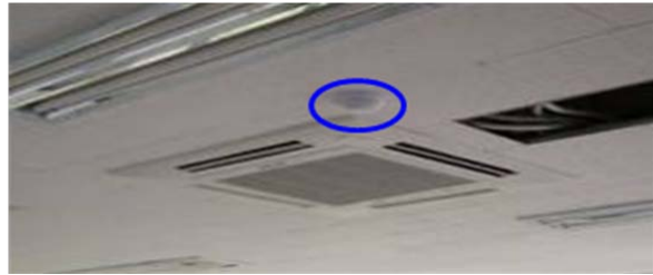
Avoid installation in the direction of discharge
