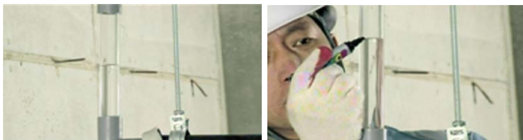
Check for leakages after 24 hours
