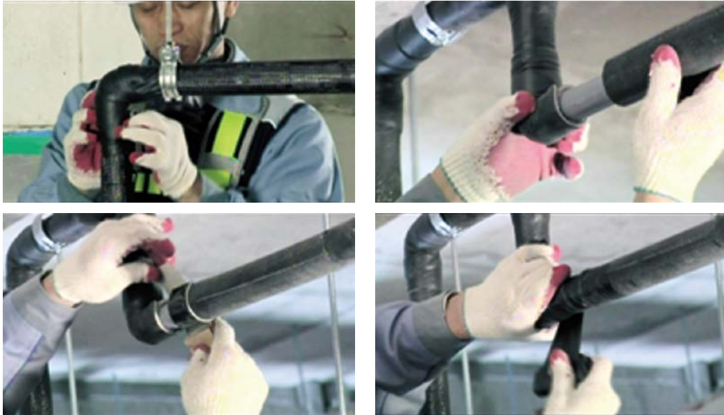
Insulating bonded/joint area of Drainpipe
