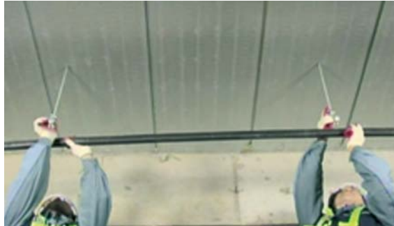
Cutting and mounting the drainpipe
