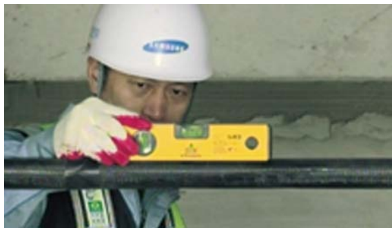
Checking the slope
