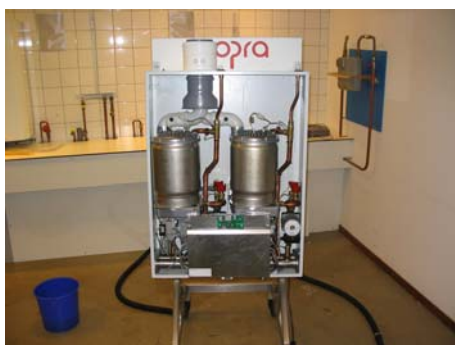
Wall hung, fan flue, room sealed, high efficiency gas boiler
